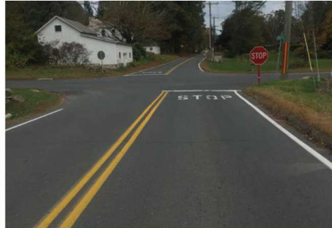
Talmadge Hill Rd/Matthew Rd/ CT-68 (Cheshire Rd)
